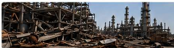
The explosion caused extensive damage to the Isomerization Unit and surrounding process units.
